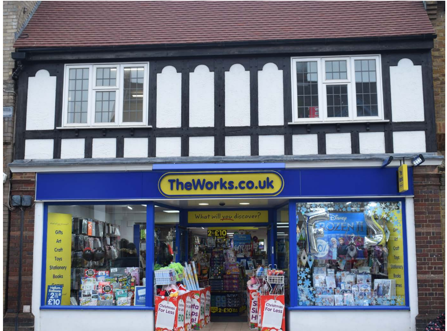
Frontage is not sympathetic to the character of the building. Bright colours detract from the historical aesthetic.
